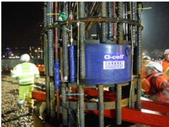
Thermal cables with O-cell assembly
